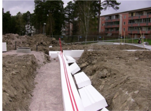
Fig. 2.5 Pipes in EPS blocks
