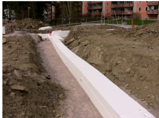
Fig. 2.6 Top half of EPS blocks
