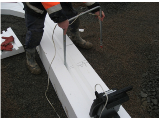
Fig. 2.4 Hot wire cutting
