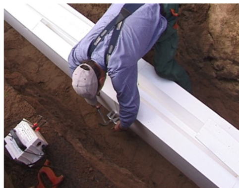
Fig. 2.3 Jointing EPS blocks
